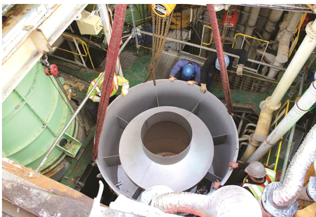
Figure 2. Rigging the scrubber section into the ship.
