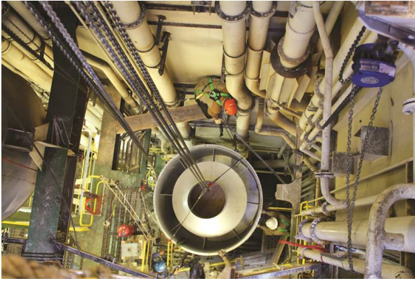
Figure 4. Lowering the scrubber section into place.
